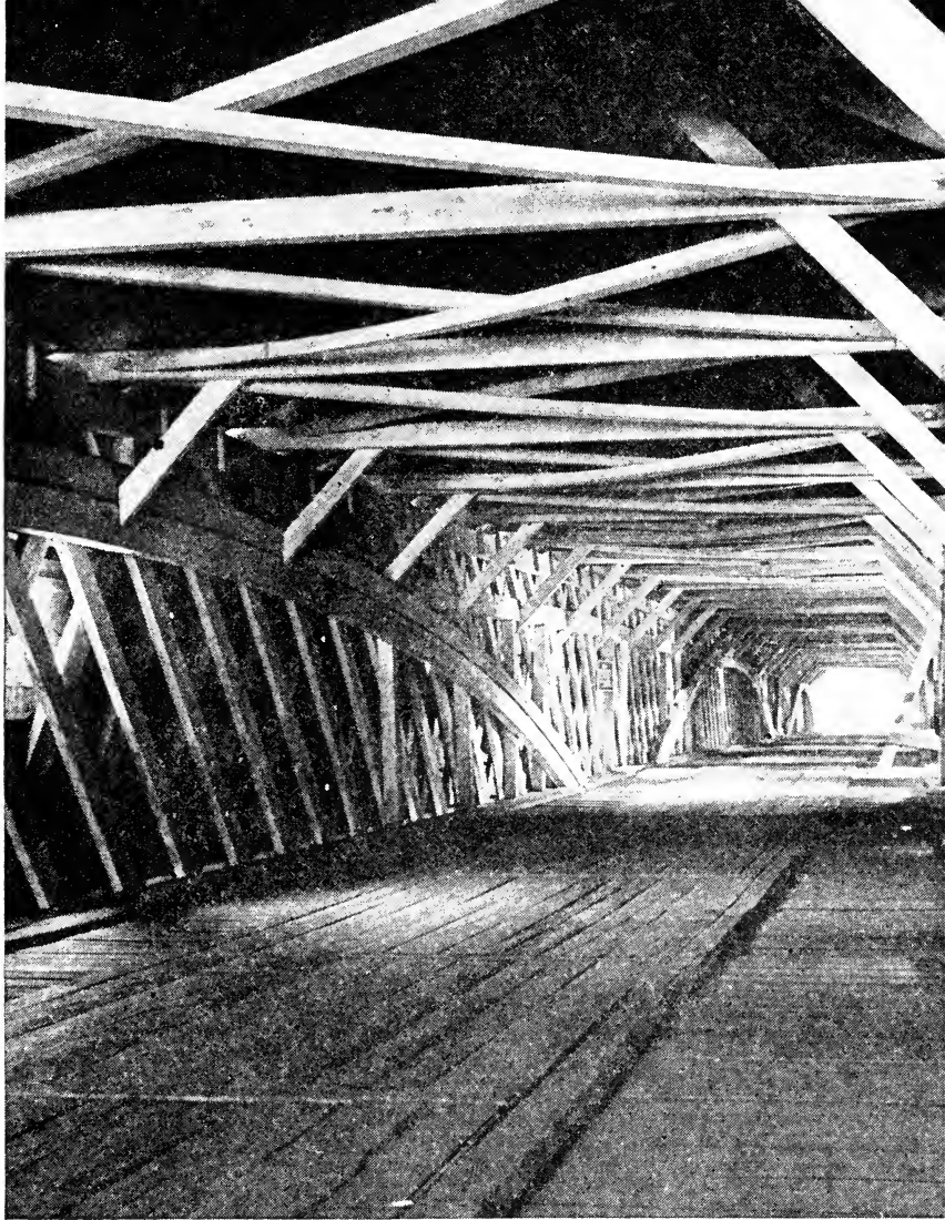
OLD COVERED BRIDGE ACROSS DELAWARE RIVER AT STOCKTON
